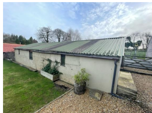
Plate 2: The Barn (Western Aspect)
