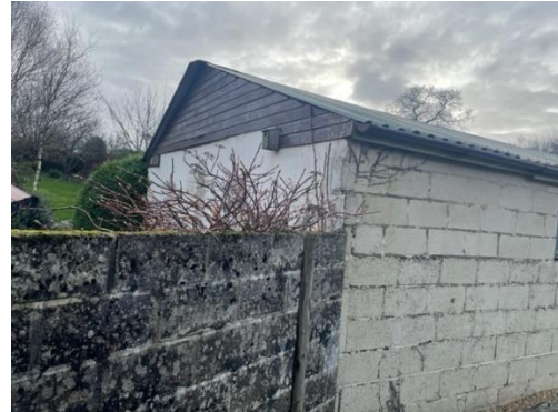
Plate 4: The Barn (Northern Aspect)
