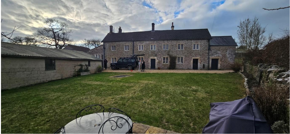
Above: Rear elevation of main house, barn on the left, access track behind wall
