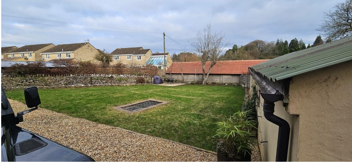
Above: Partial side elevation of barn looking towards neighbours
