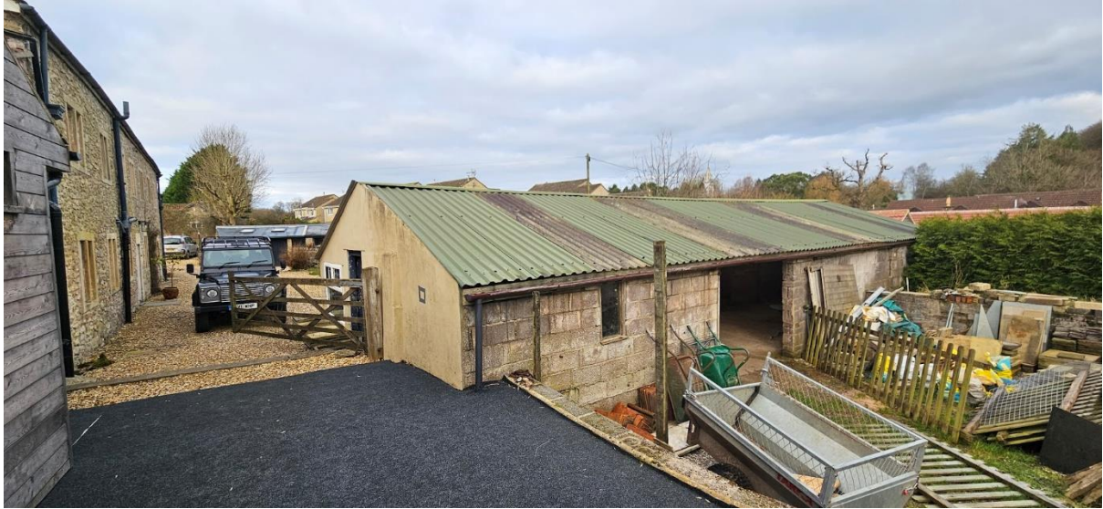
Above: Side and rear elevations of barn and partial view of rear elevation of main house
