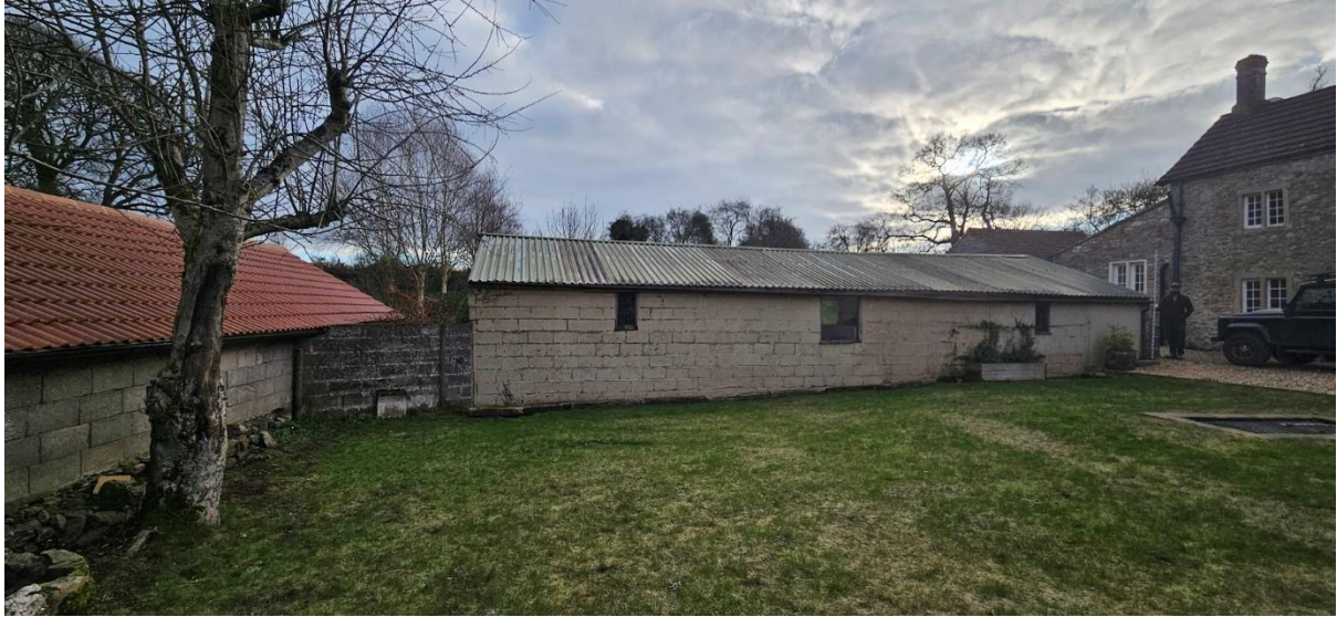
Above: Front elevation of existing barn, neighbours outbuilding/ garage to left
