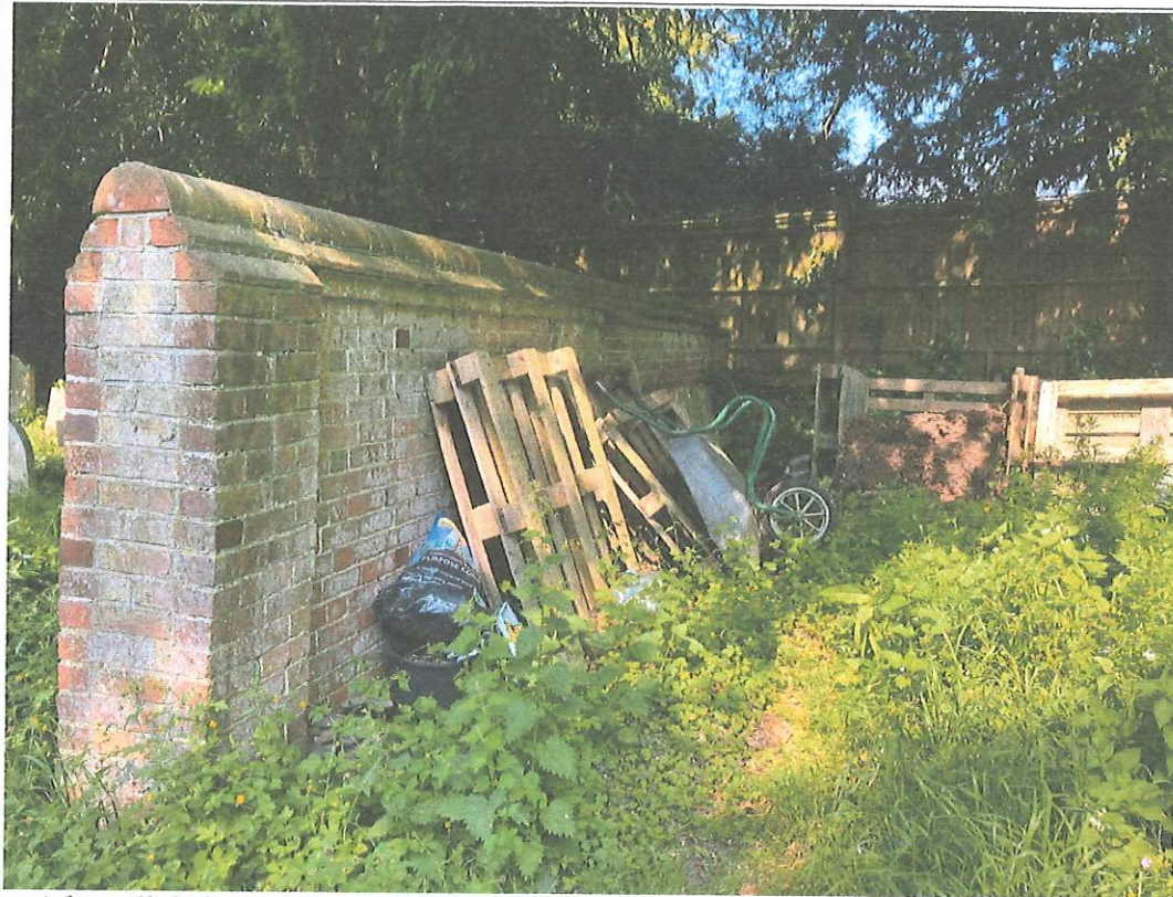
Brick wall, behind which the shed will be positioned, roughly in position of the composting bin in this photograph. The area will be tidied and wheelbarrow stored within the shed.
