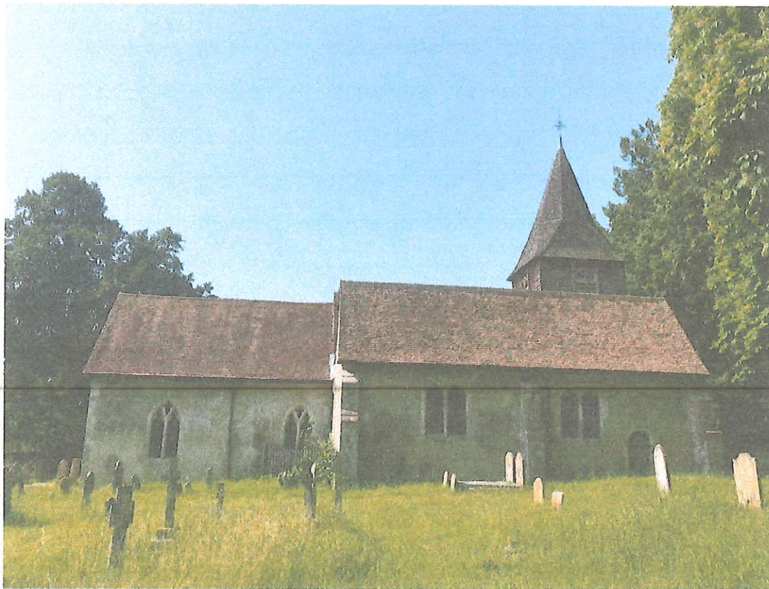
North side of the church building, as seen from the churchyard.
