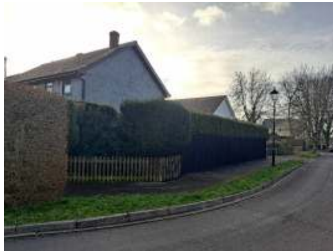
View of the west elevation, including boundary and highway
