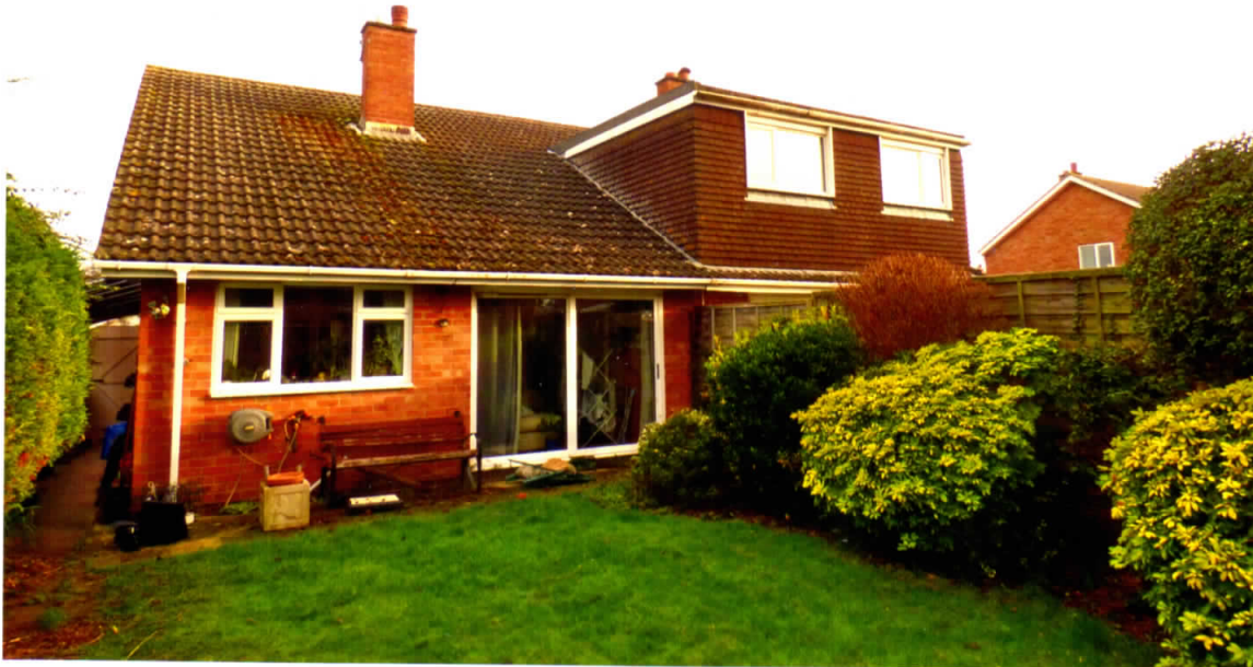
3. View of gable wall at No.92
