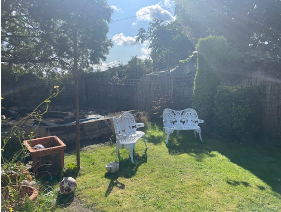
Above : The rear garden – the new building will be located on the site of a previous outhouse and since demolished. The foundation slab and some brickwork remains.
