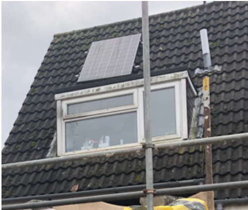
Original Dormer Main Bathroom – Old Window
