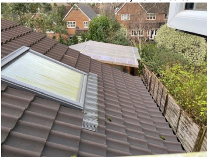
Roof view of Gable end by Main Bathroom.
