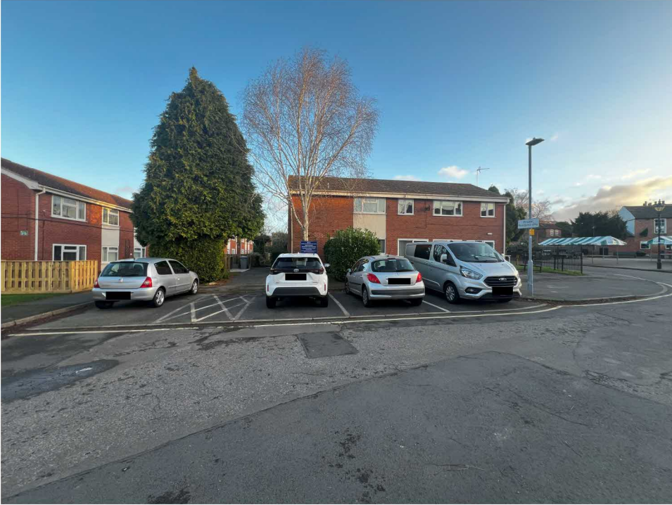
Existing parking at the front of the building
