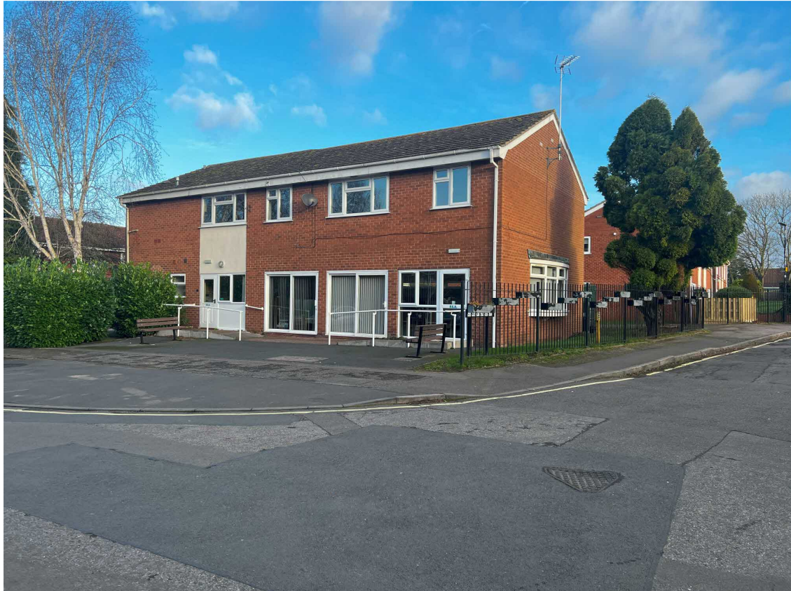
View of the existing front and side elevation
