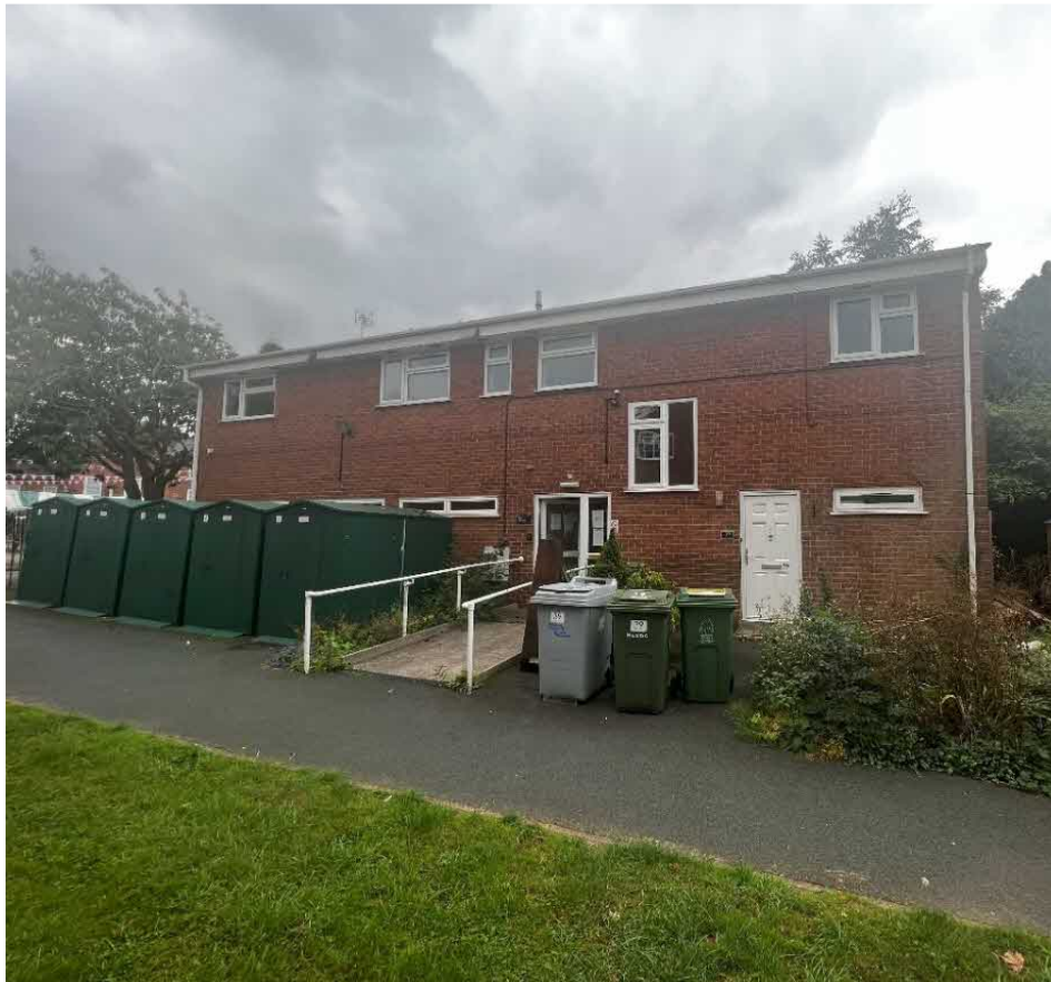
Rear Elevation photo
