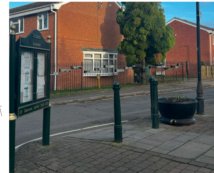
Block paving and bollards to match existing at Market Square located opposite
