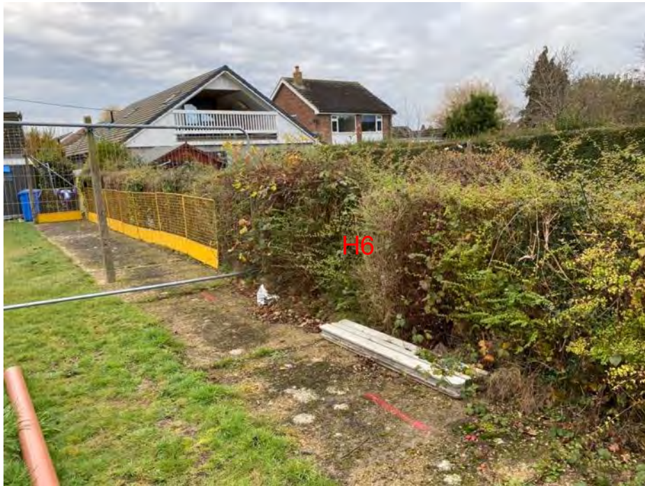
Photoview 5: View looking south along H6.
