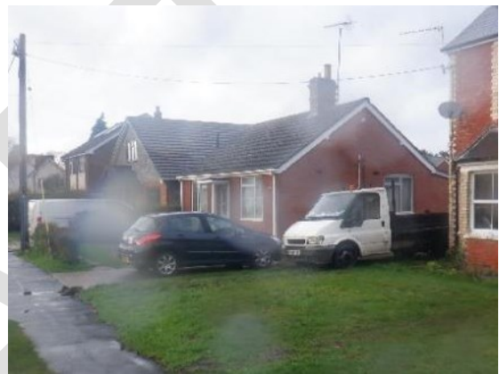
10. Woodside residential property viewed from the southern elevation (B2).
