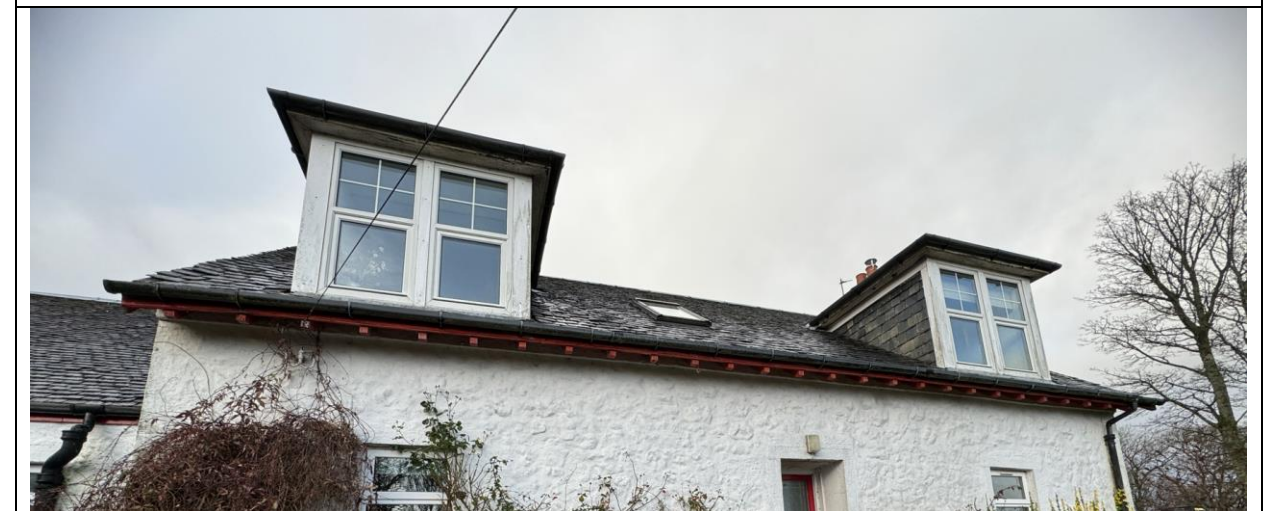
Figure 6 Images of external roof showing slate covering, eaves, dormers and metalworks
