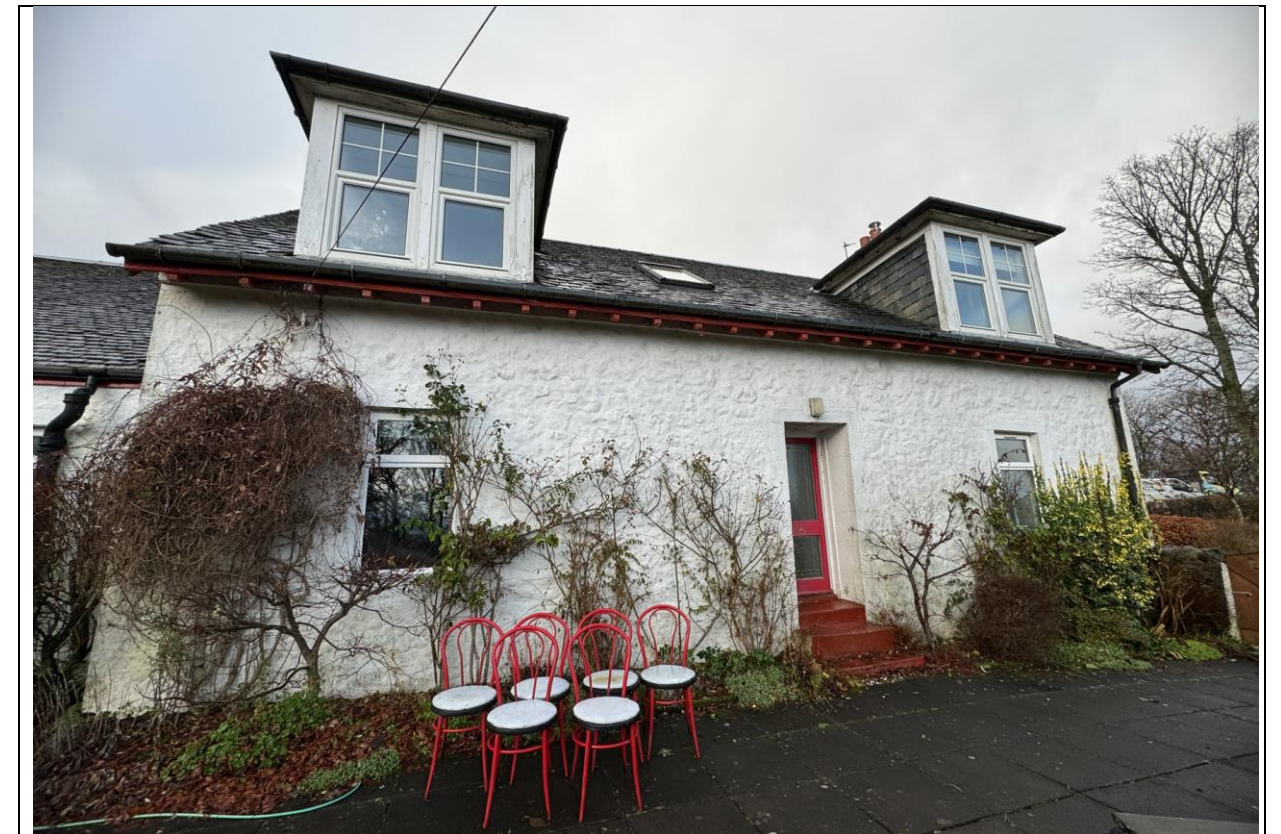
Figure 3 Image of elevation facing away from courtyard
