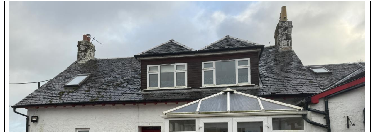
Figure 5 Images of external roof showing slate covering, dormers, chimneys and metalworks
