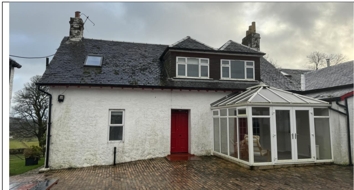
Figure 2 Image of elevation facing courtyard
