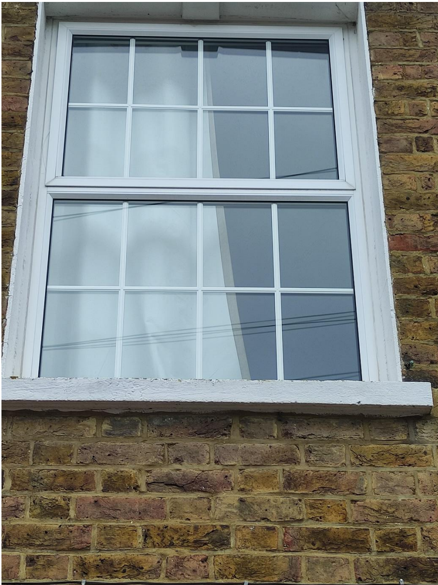
Front bedroom window left:
