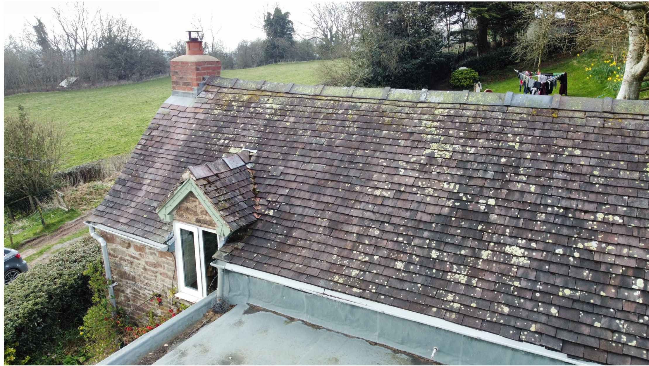
Reclaimed Plain Tile to Match the Existing Roof
