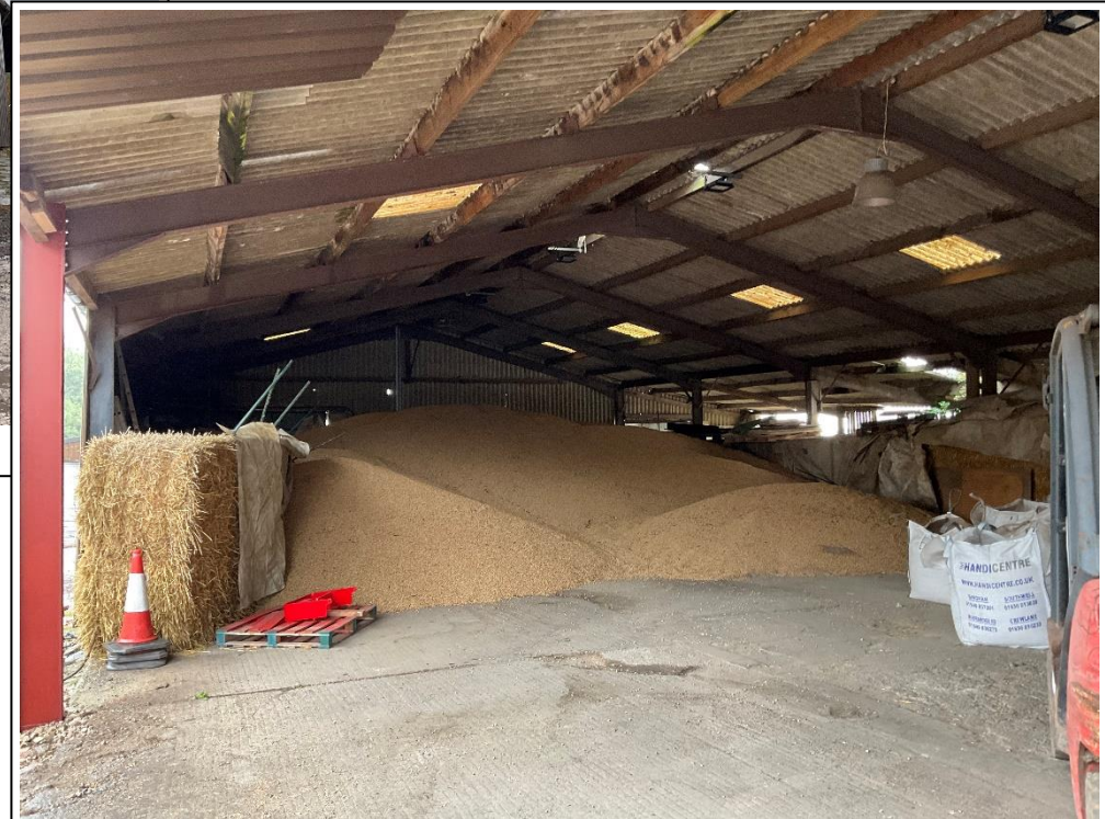
2.- General internal view
