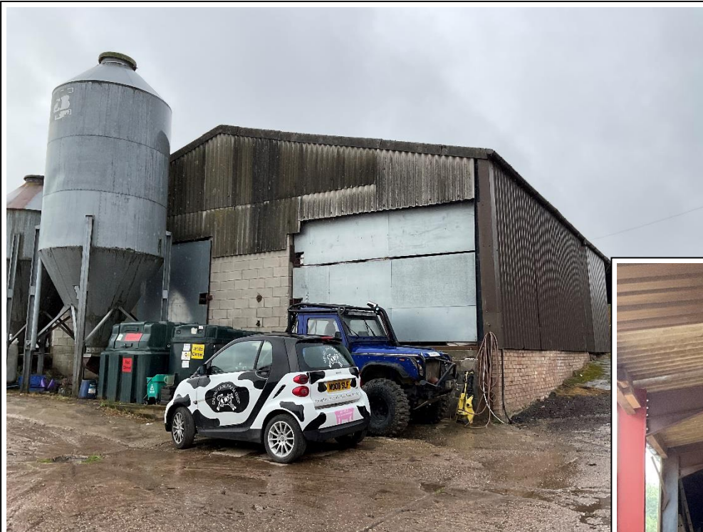
1.- General view from rear left
