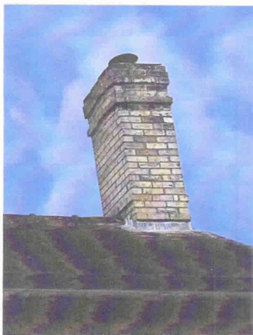
front RH side chimney
