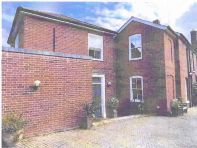
rear extension brickwork
