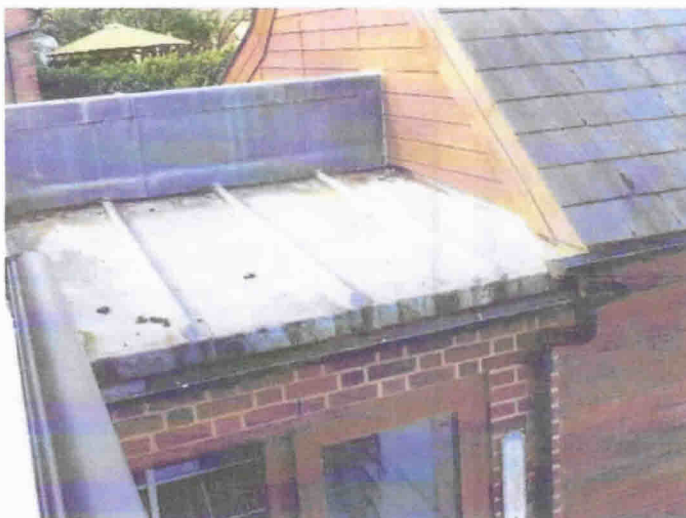
lead roof over link
