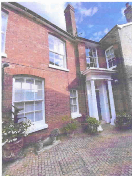
mid section LH side chimney (note window below)
