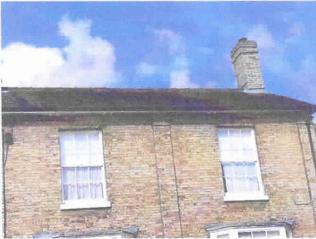
main front roof slope
