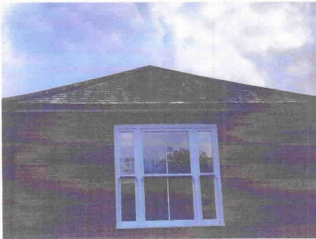
rear extension roof covering
