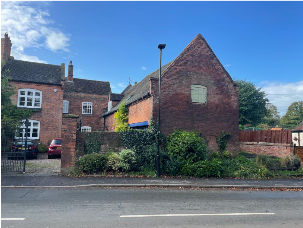
Figure 2 – This photo shows the relationship between the Former Stables and Elswick House.
