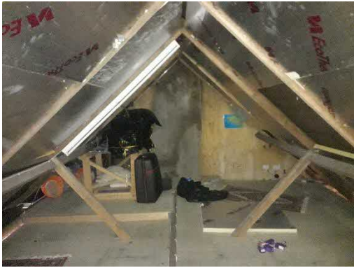
Figure 3 Roof void in Bedevire
