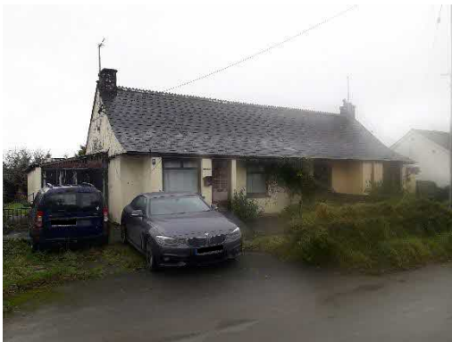
Figure 1 East side of the building
