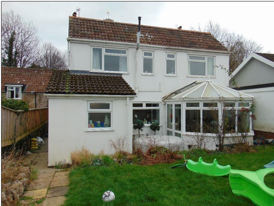
Above: the rear of the dwelling showing the utility room / bathroom extension on the left and the conservatory on the right
