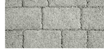
Permeable paving, example
