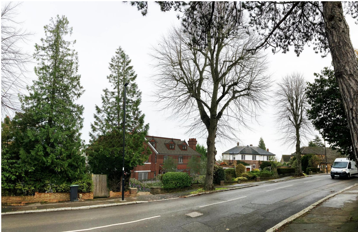
Figure 10: Proposed View 2 looking north-eastward along Crescent East towards the Hadley Wood Conservation Area.
