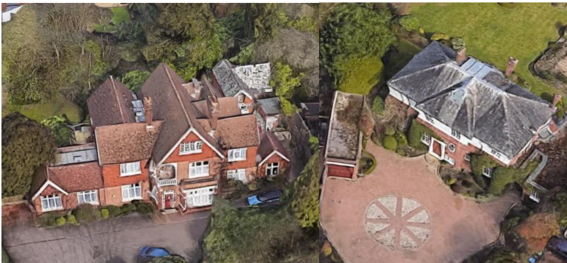
Figure 8—The two neighboring properties. No. 21 and no. 25
