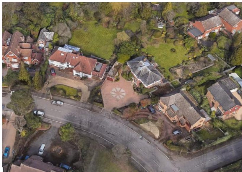
Figure 5 – transition of no. 23 and 25 Crescent East. Note the awkward location of no. 23 relative to no. 25.
