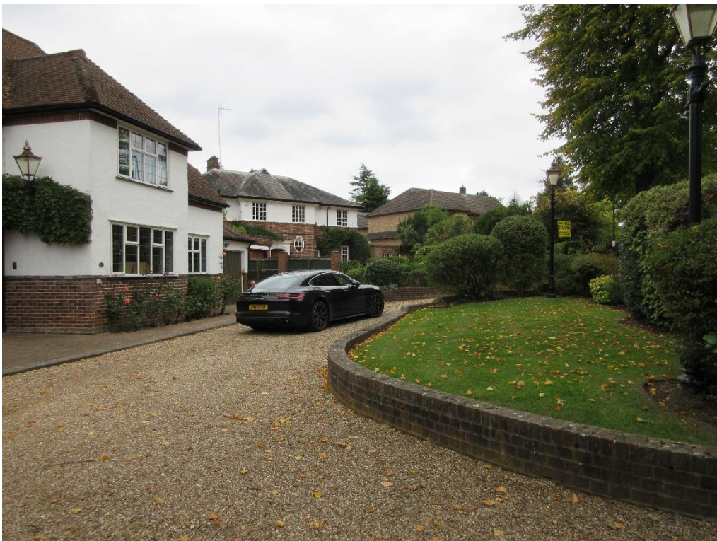
Figure 18: Front elevation of no. 23 Crescent East, and no. 25 to east.
