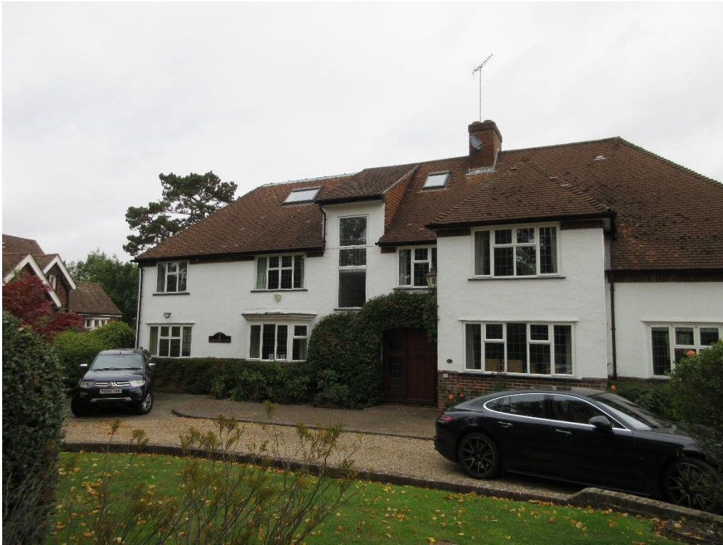
Figure 36: Front elevation of no. 23 Crescent East – west side.
