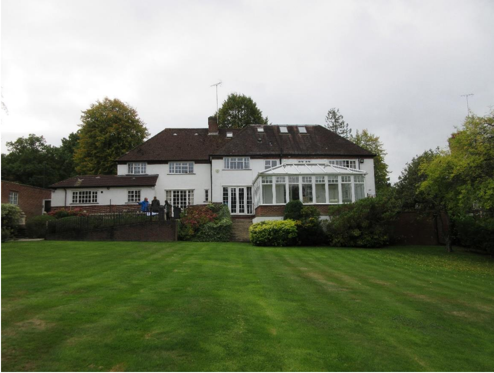
Figure 40: Rear (north) elevation of no. 23 Crescent East.
