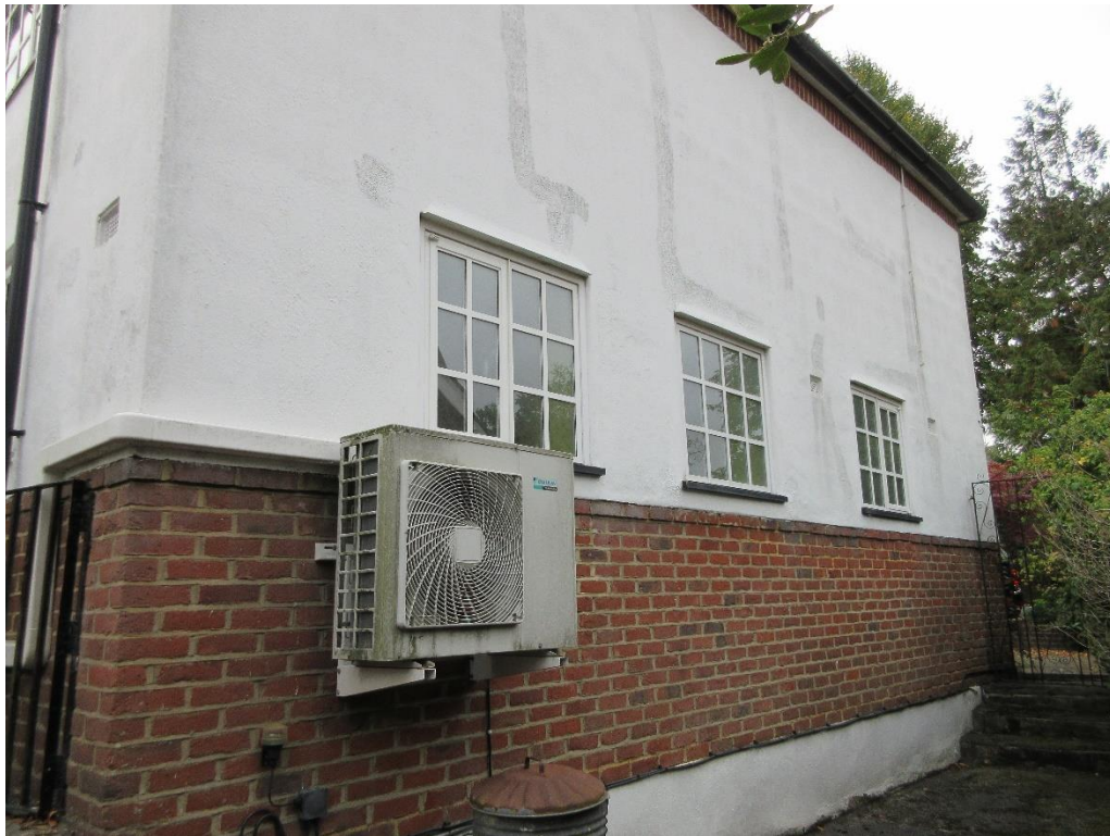
Figure 38: West elevation (front part) of no. 23 Crescent East.
