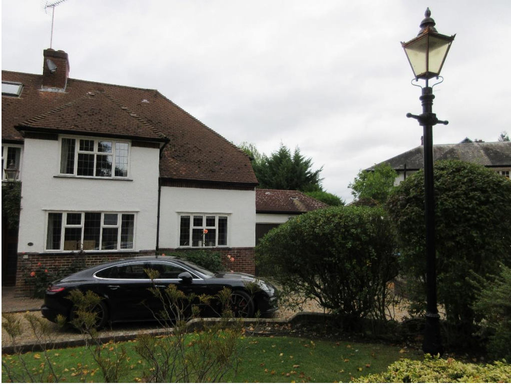
Figure 37: Front elevation of no. 23 Crescent East – east side.
