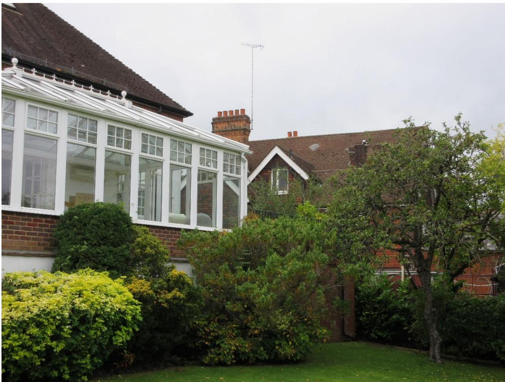
Figure 15: Rear (north) elevation of no.s 23 Crescent East, with no. 21 on the right.
