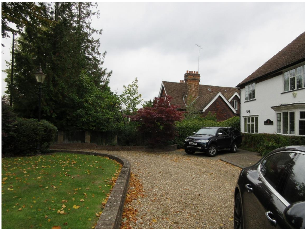
Figure 13: Front elevation of no. 23 Crescent East, and no. 21 to west.
