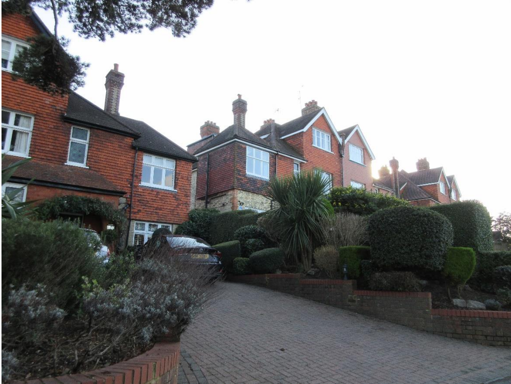
Figure 3: No.s 39, 41 & 43, and 45 & 47 Crescent West.
