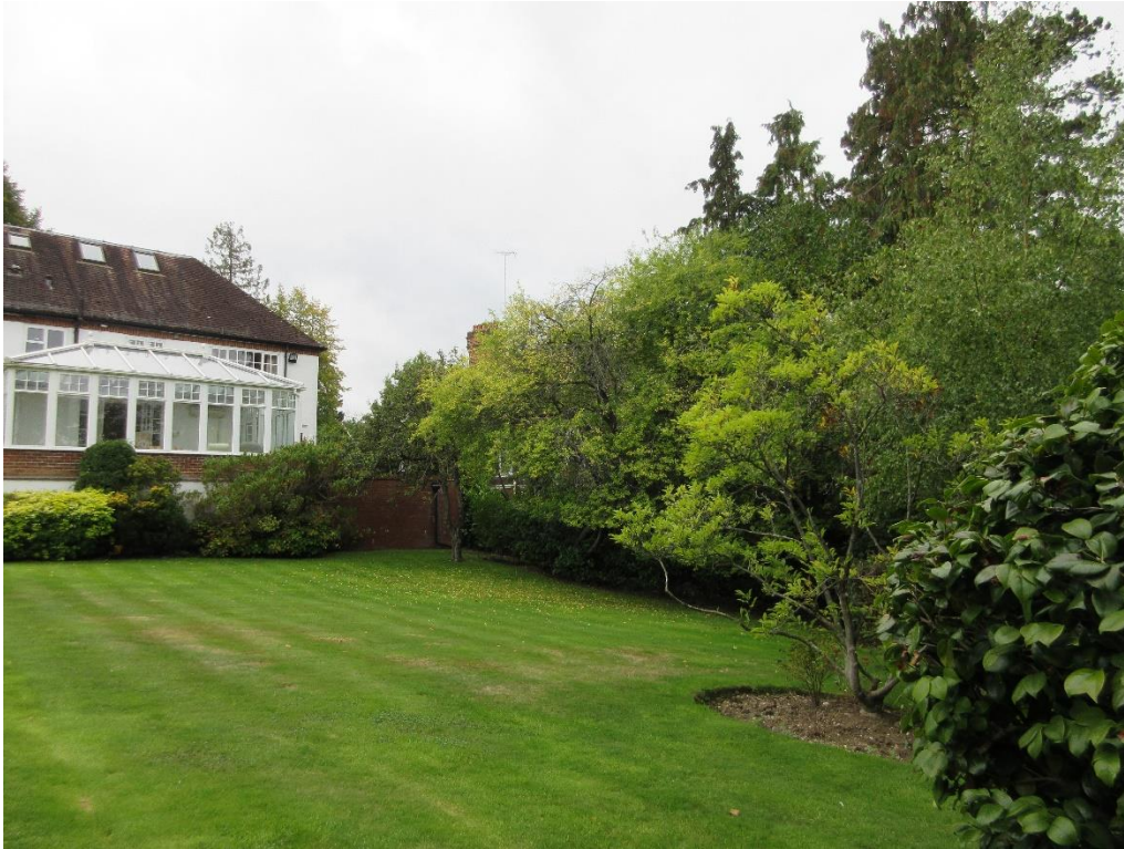
Figure 14: Rear (north) elevation of no.s 23 Crescent East, with no. 21 on the right.
