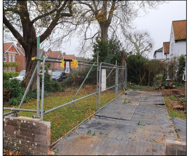
GP2: Tree protection barriers & trackmat ground protection
