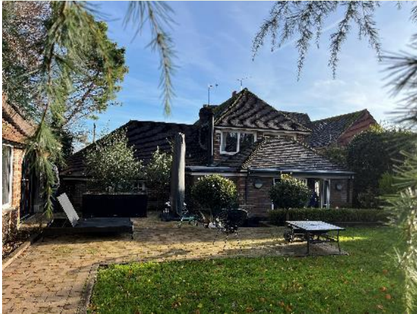
Rear of the Assessed Structure Western orientation
