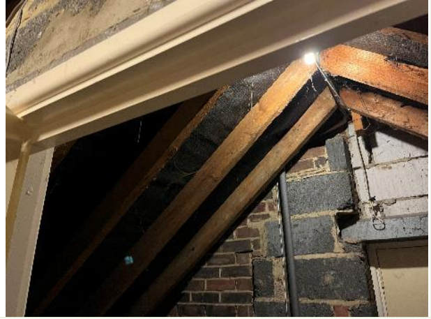
Some of the loft voids are accessible. The areas that are accessible are all lined with bitumen felt. No evidence of bat roosting or bird nesting was found
