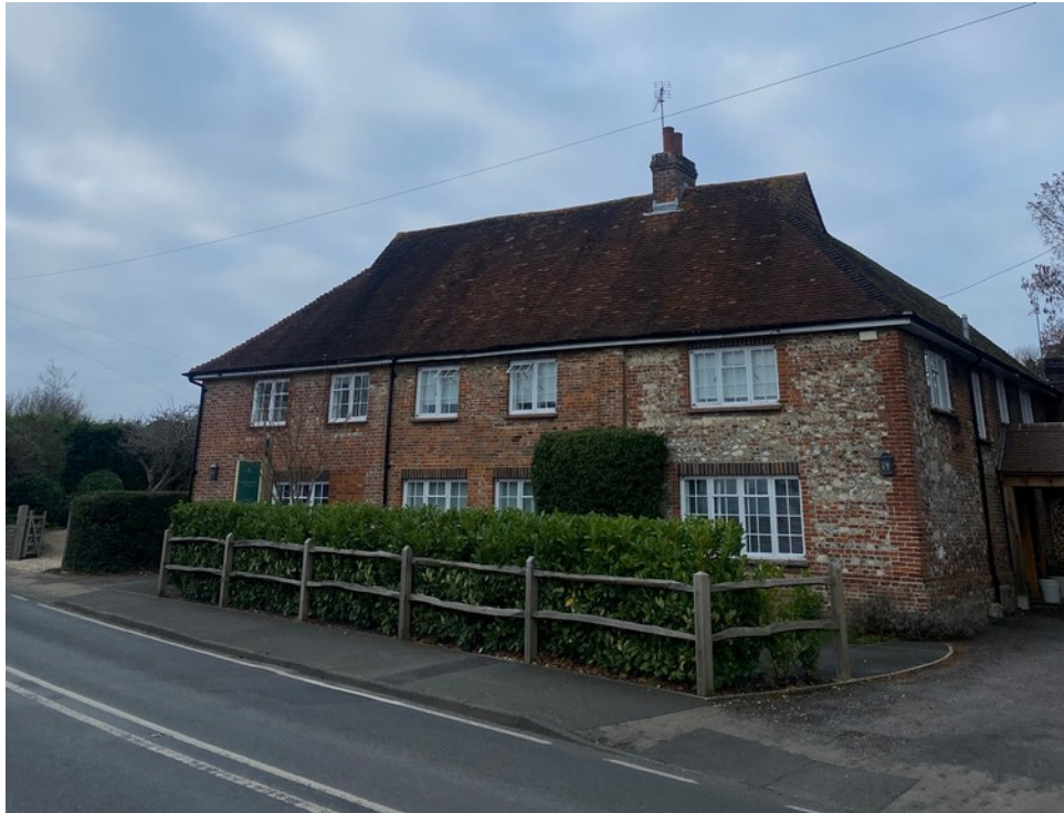
Image 1: Showing the front of the property
