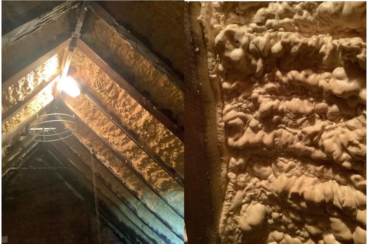
Photo 1 – Inside of the loft showing the existing spray foam insulation.
