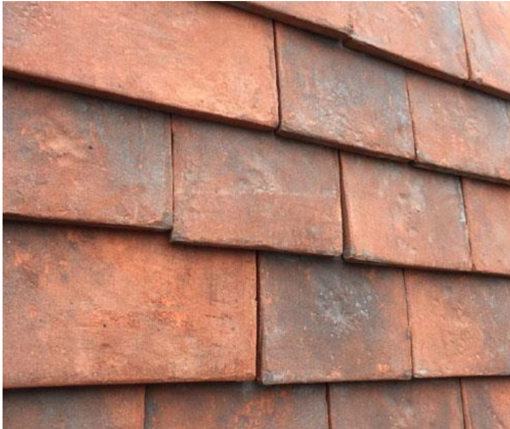
Conservation Weathered clay tile
