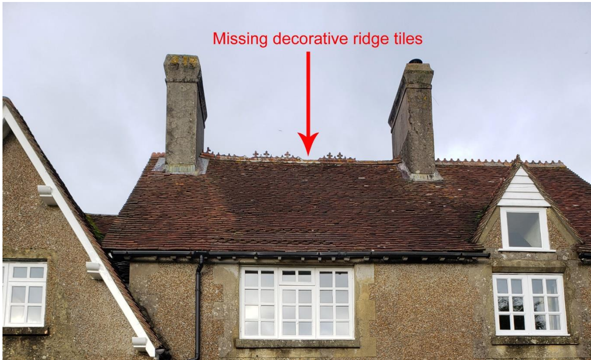
Photo 4 – Rear elevation roof
