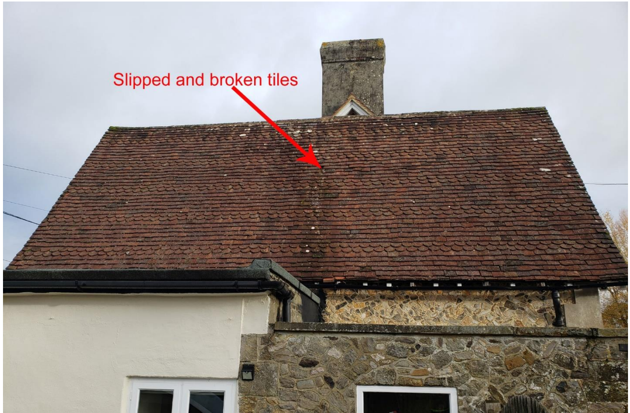
Photo 5 – Right elevation roof
