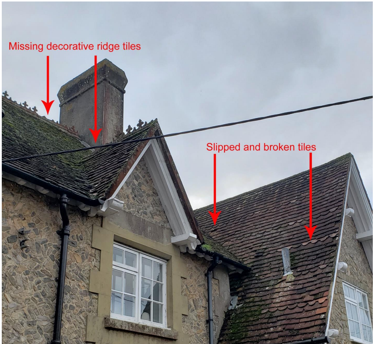
Photo 2 – Front right elevation
