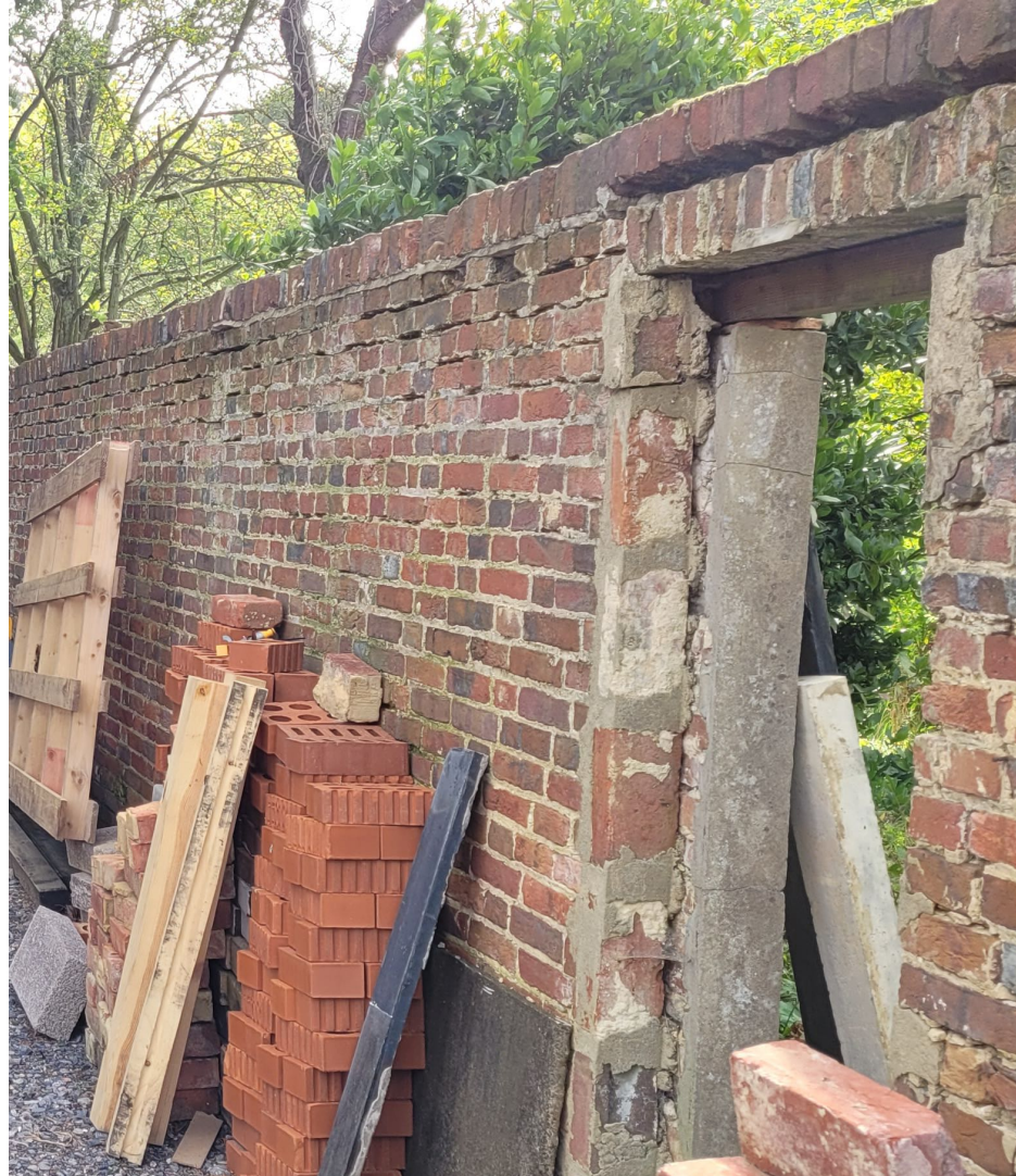
EXISTING LISTED GARDEN WALL
