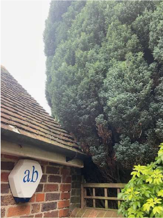
Photo 4. T1 touching roof of Parish Council Offices.
