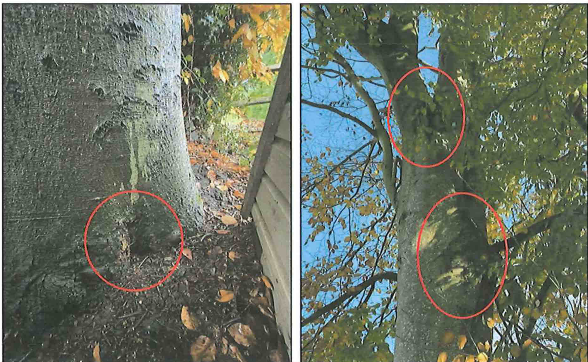
Fig.2 - western buttress root and fabric of outbuilding 18cm apart, the moribund bark area is circled red
