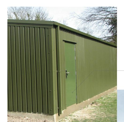
Proposed steel personnel doors Proposed insulated cladding to be finished in olive green
