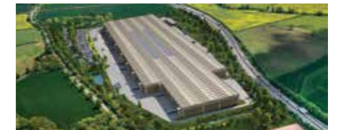
Primark Distribution Centre Kettering, England UK
