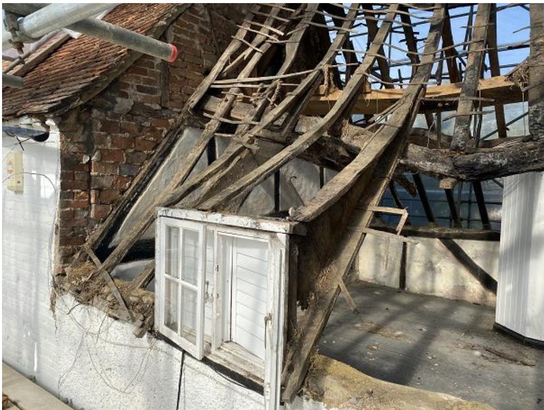
Plate 10: South-facing roof slope looking north, showing construction of westerly dormer
