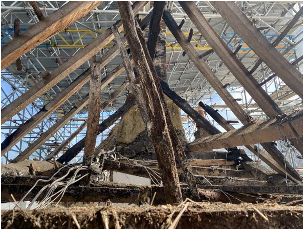
Plate 12: View looking east of underside of roof structure in western bay
