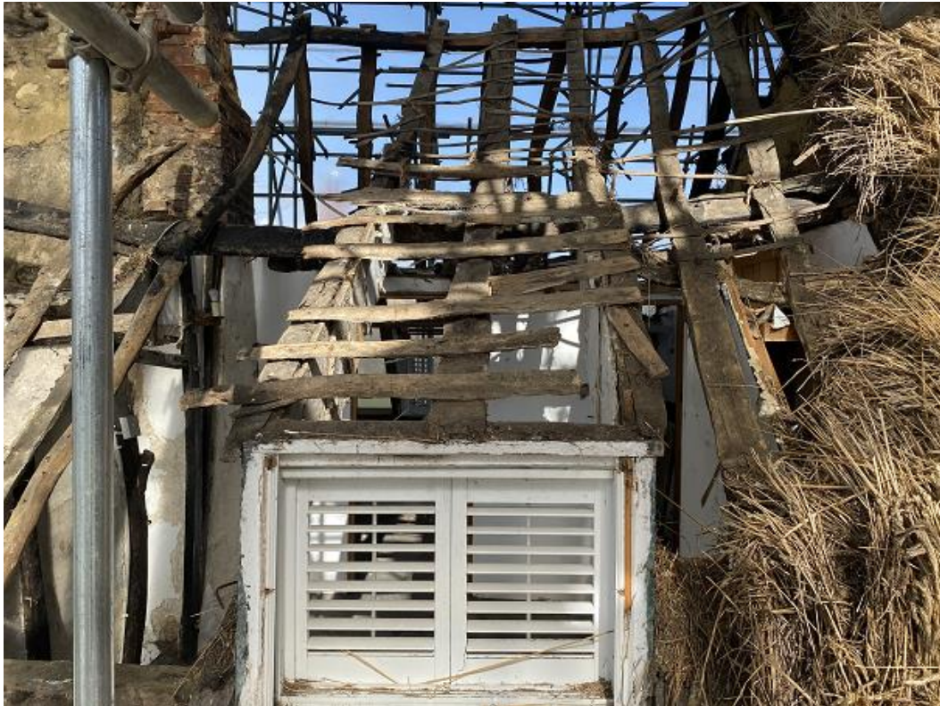
Plate 9: South-facing roof slope looking north, showing construction of easterly dormer
