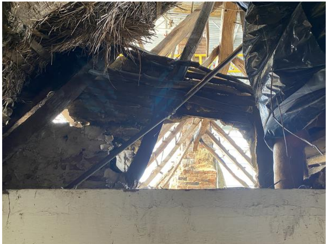
Plate 14: View looking west of rear of plastered partition
