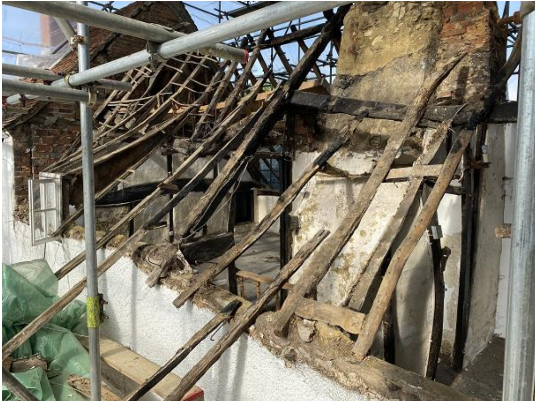
Plate 7: South-facing roof slope looking west
