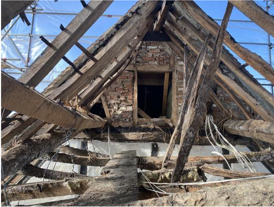
Plate 11: View looking west of underside of roof structure in western bay
