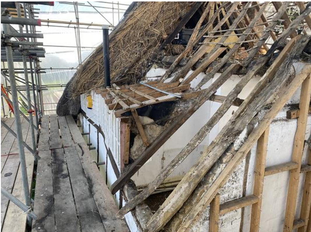
Plate 6: North-facing roof slope looking east, showing modern dormer construction
