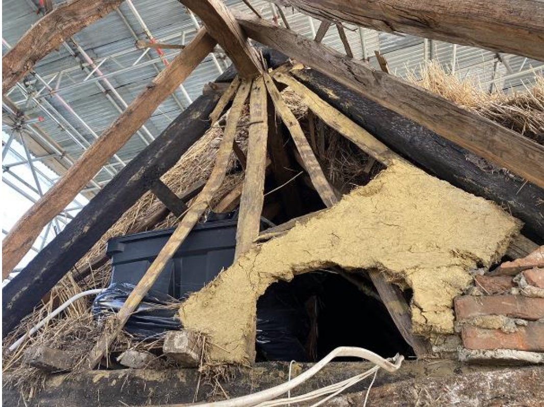
Plate 13: View looking east of plastered partition at east end
