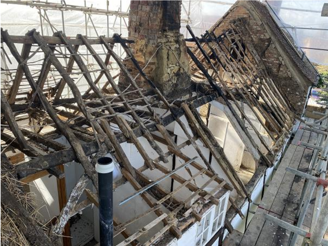
Plate 1: North-facing roof slope looking west
