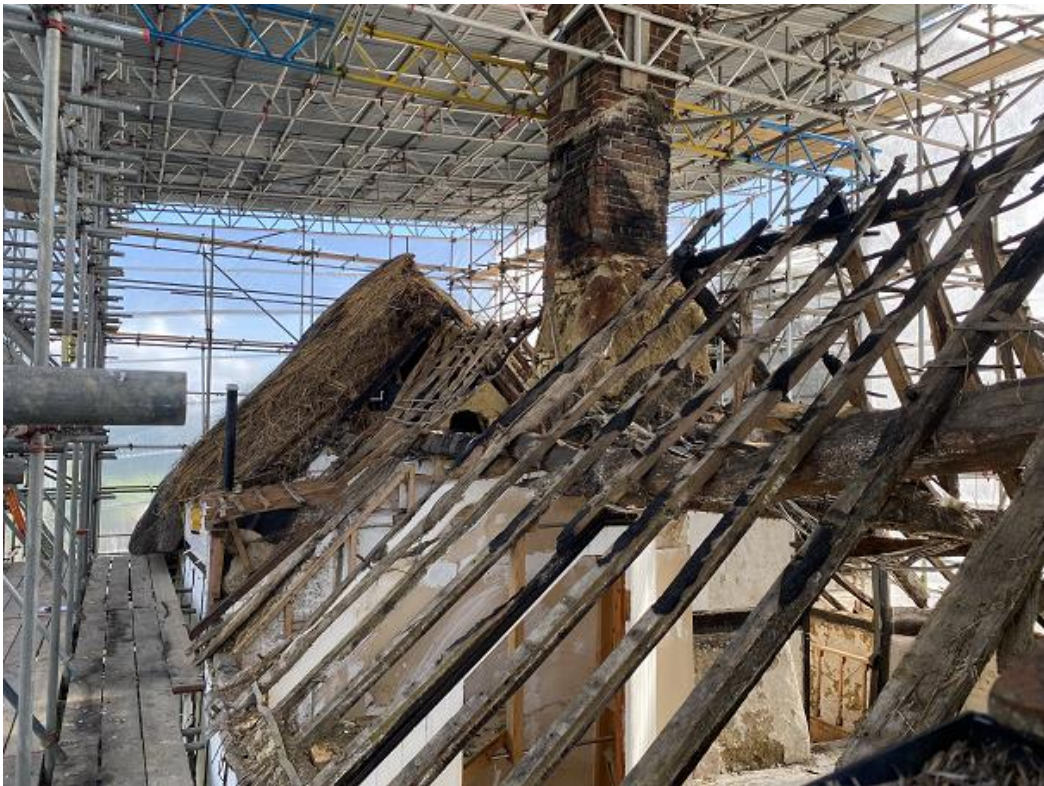
Plate 2: North-facing roof slope looking east
