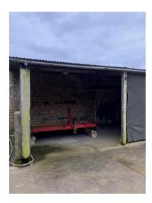
This building has 2 sections, the older part is stone which has been partly rendered internally presumably when livestock pens were installed. The roof is monopitch on a timber frame with tin sheeted covering. The lean to is timber framed, with a similar roof. The stone walls appear sound but in need of localised repair and repointing. The timber sections are in good order.
