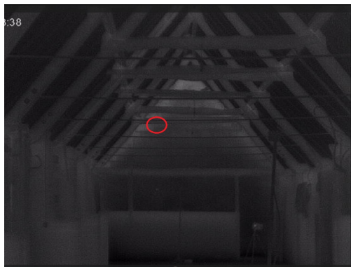
Figure 3. Roost 3; behind beam on northern gable wall of Building E.
