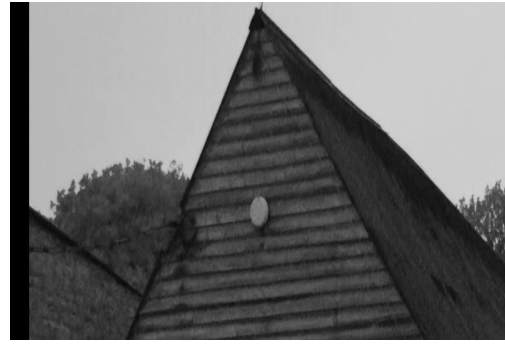
Figure 2. Roost 2; cladding on south gable wall of Building E.
