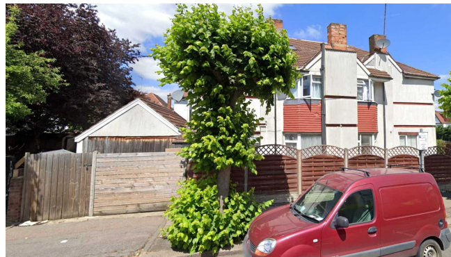
EXISTING BUILDING - GAINSBOROUGH GARDENS VIEW
