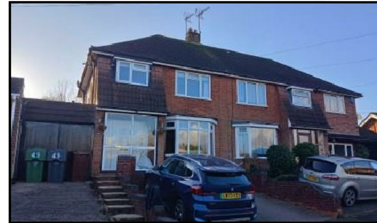
FRONT ELEVATION PHOTOGRAPH
