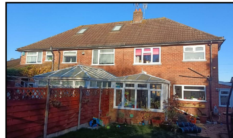
REAR ELEVATION PHOTOGRAPH
