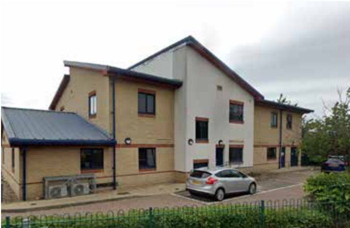
Rowner heath centre - Brick and angled metal roofs
