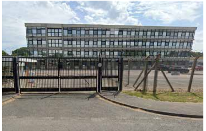
Glazed frontage of the Centurion Building
