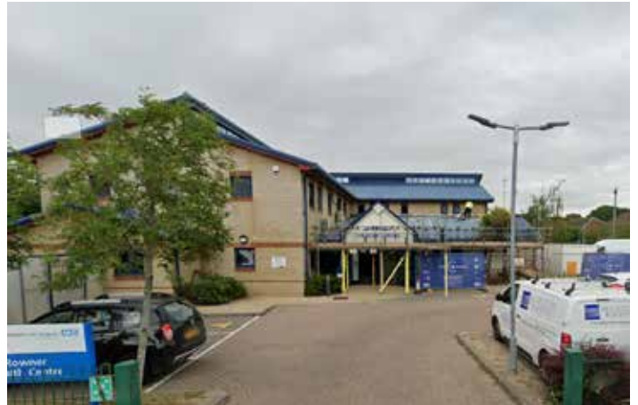
Rowner heath centre - Brick and angled metal roofs with rooflights
