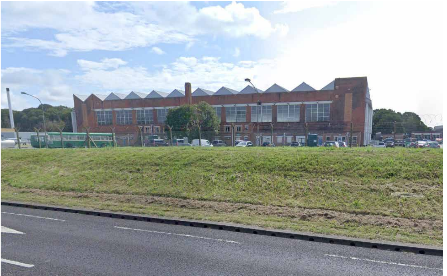
HMS Sultan - pitched roof form to allow light deep into floor plan
