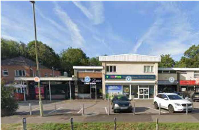
Retail units off Rowner Road
