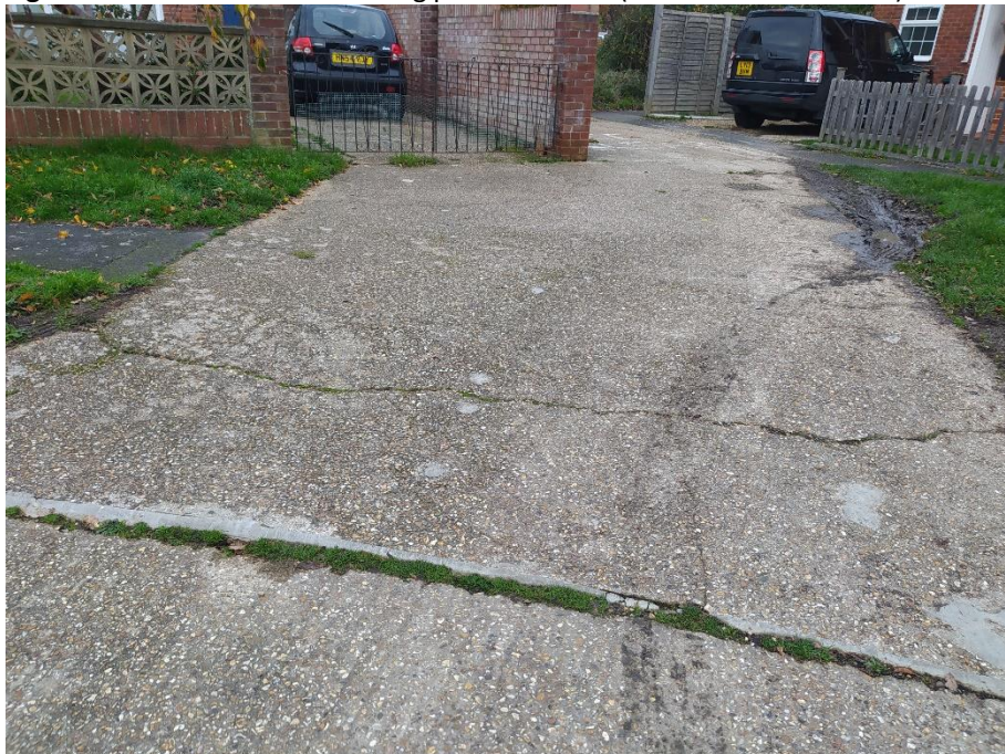
Figure 8. View of the hard standing present on site (taken November 2023).
