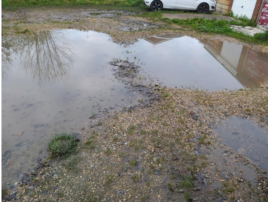
Figure 7. View of the area of gravel present on site (taken November 2023).
