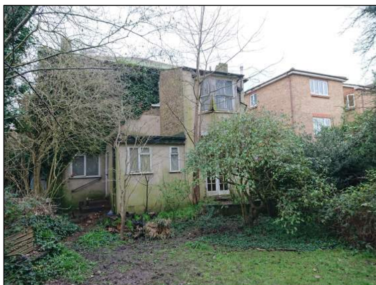
Figure 3.2 Photo of the rear garden
