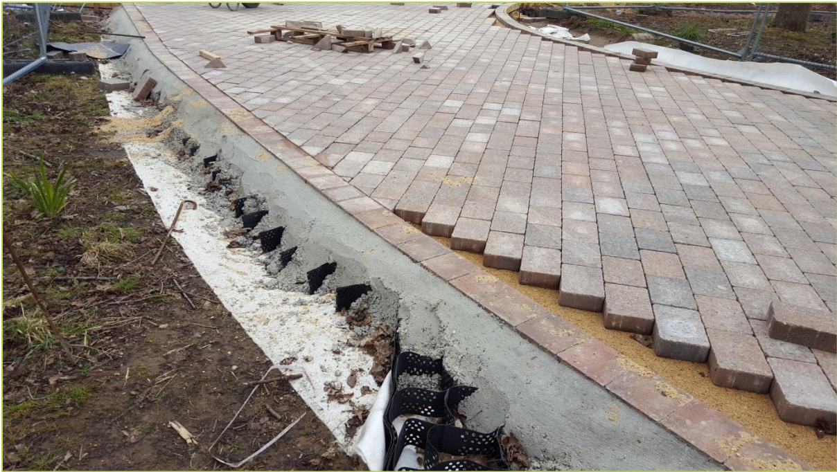
Photograph of Installed 'Reduced-dig' 3D webbing system ground protection
