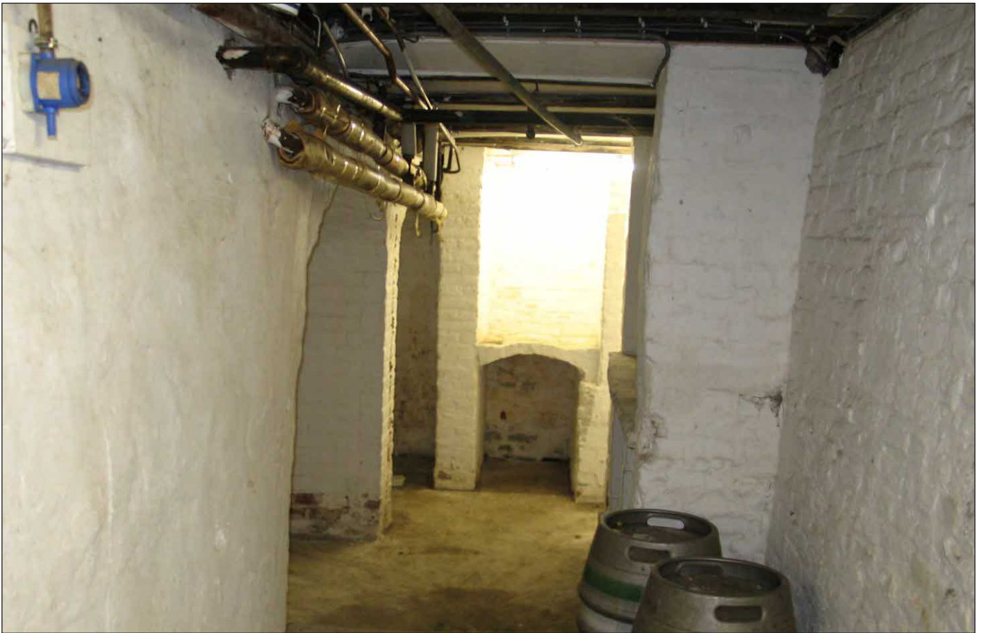
Fig 14 Upper - Cellar area Lower - Cellar Area right
