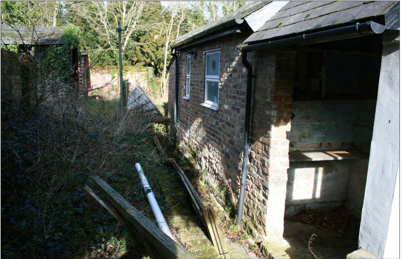
Fig 8.1 Upper - 28 Winhill toilet block Lower - 28 Winhill, toilet block west elevation
