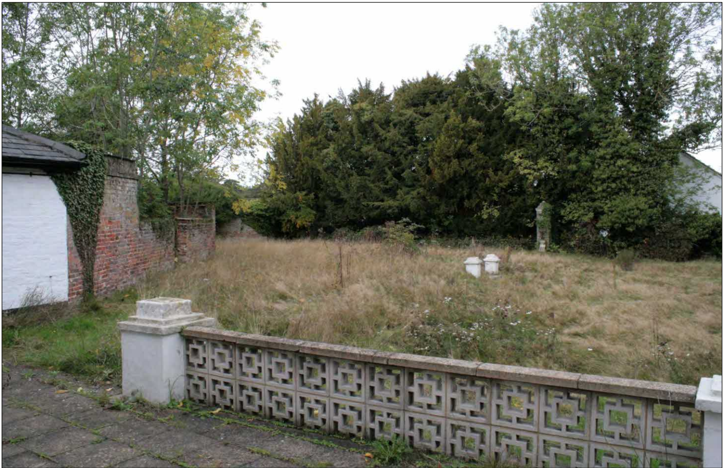
Fig 8.2 Upper - 28 Winhill toilet block, east elevation Lower - 28 Winhill, location of proposed pool house
