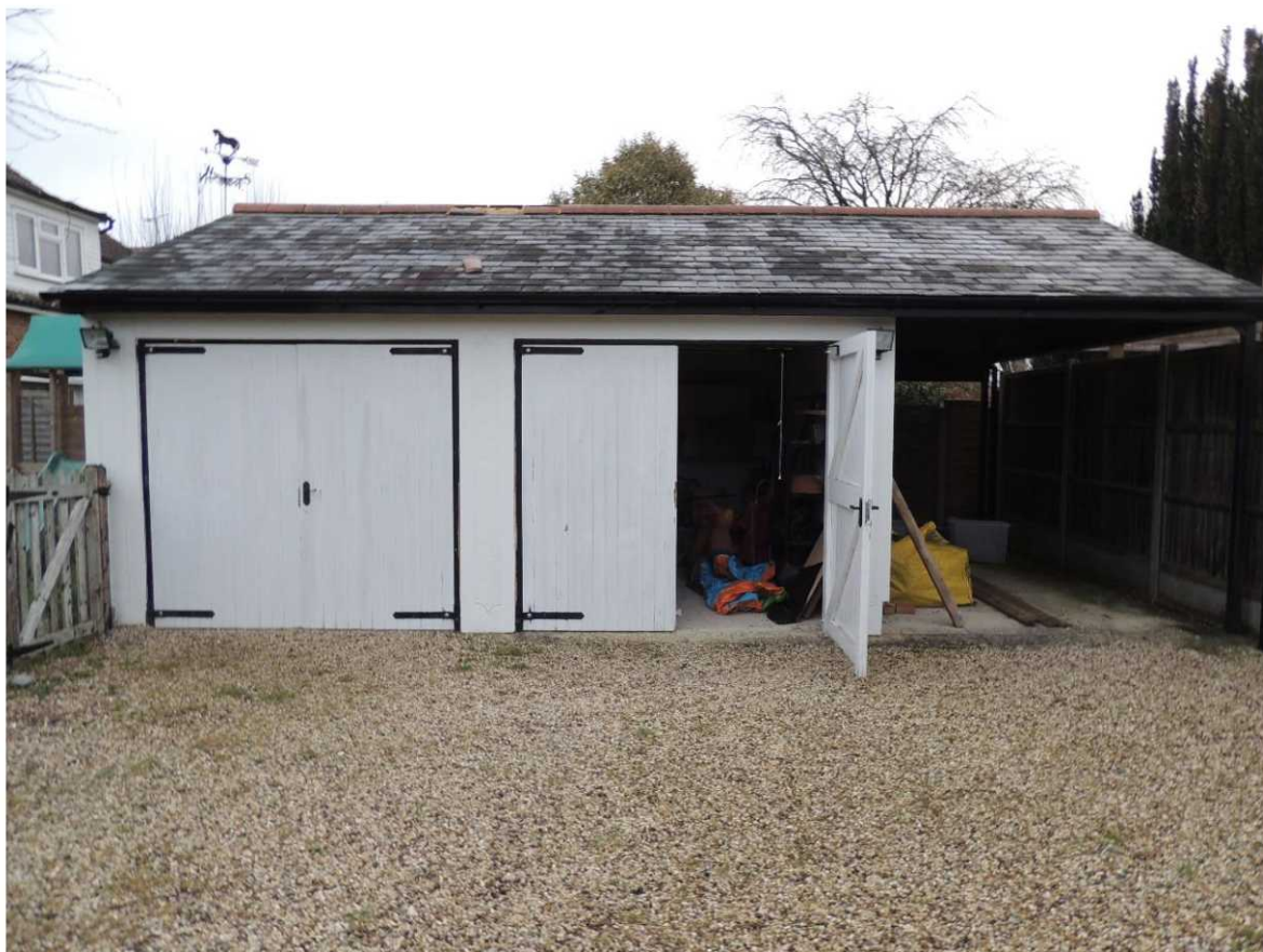
Photo 1: Western elevation. The proposal is to convert to an annexe
