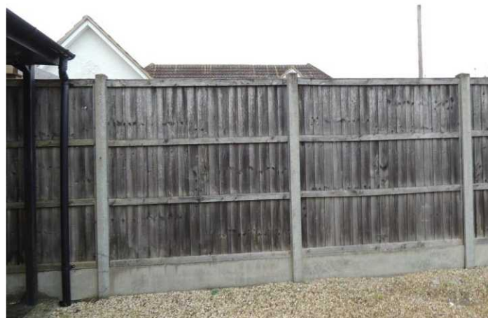
Photo 12: Southern boundary with housing beyond
