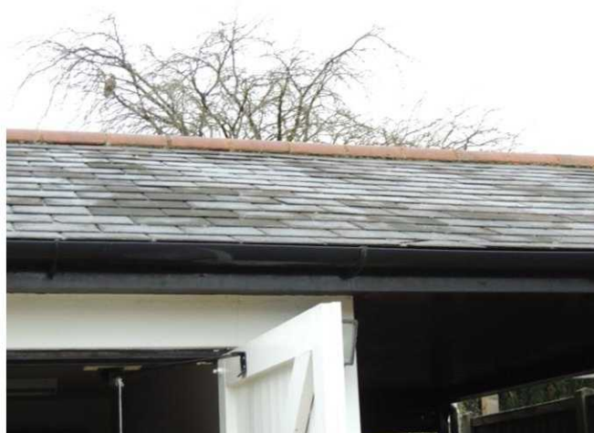
Photo 8: Note tight seal to roof slates
