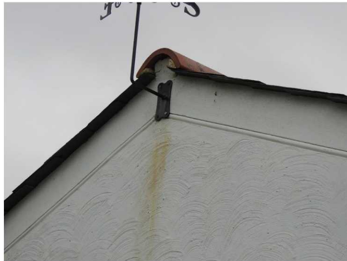
Photo 6: Note tight seal to gable
