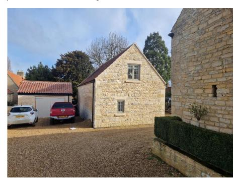
To the south-east of the site, a new build outbuilding has been constructed. This is a one and half storey structure, constructed in a typical linear gable ended roof, in walling stone and clay pantiles. It has been confirmed that an original structure was sited in this position and the building was converted/rebuilt into its current form.
