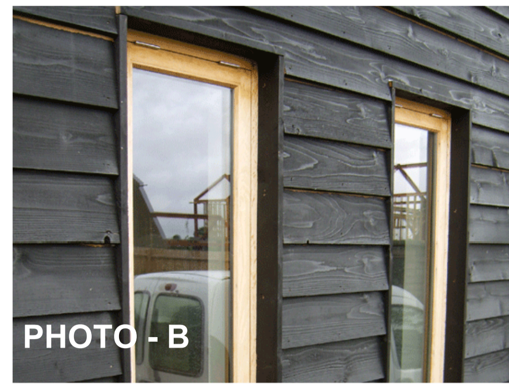
Fibre cement wood effect planking with co-ordinated black metal trims proposed instead of painted timber
