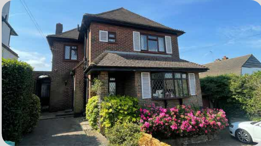
10 St Marys Road, Benfleet Essex SS7 1NR - Front View
