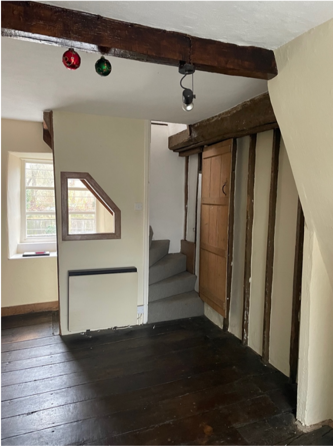
First to second floor staircase:
