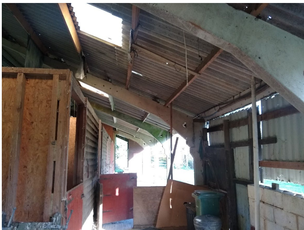
Photo 7 – East Elevation Structure.
