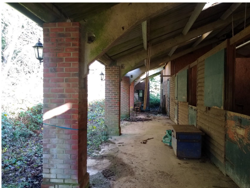
Photo 4 – West Elevations Structure.
