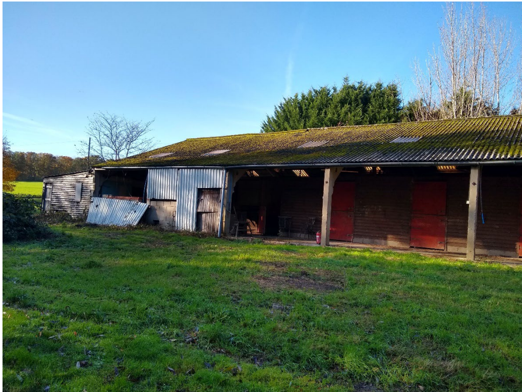
Photo 5 – East Elevation – southern end.
