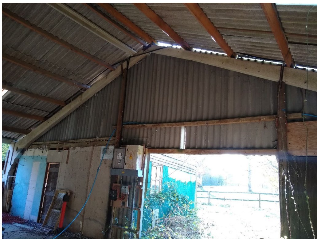
Photo 8 – Southern wall - internal.
