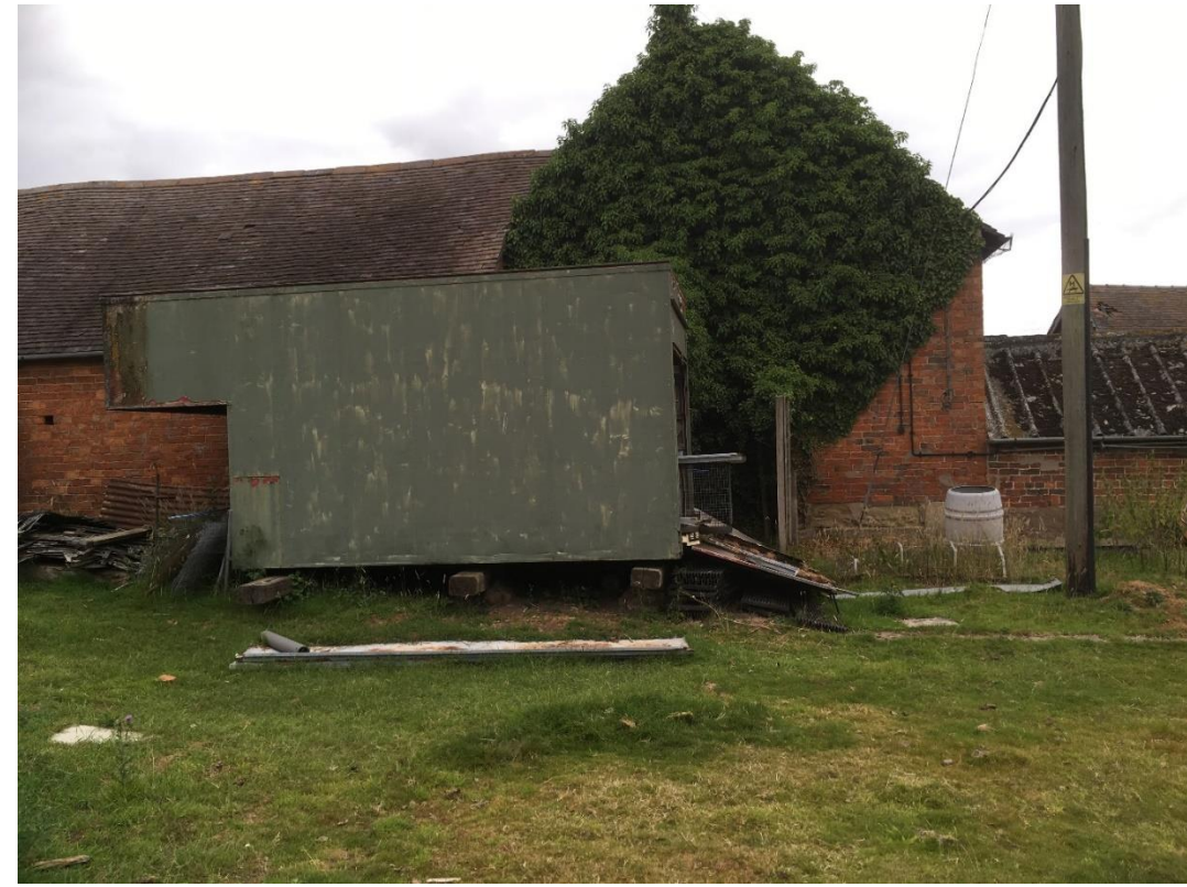
Barn B1 – Threshing Barn (side south elevation)
